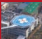
ALUMINUM HELIPORT Numazu City Hospital
